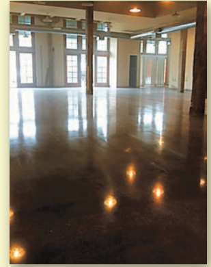
The completed polished floor is ready for customers.
