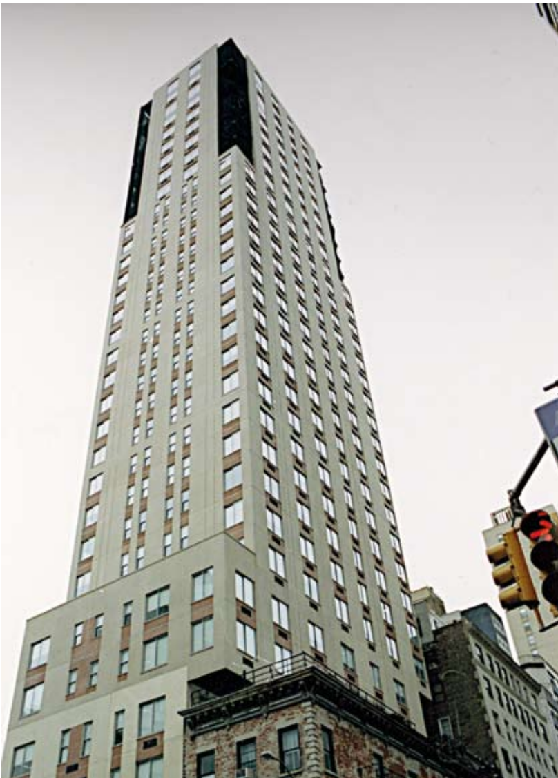
The Marriott Execustay, in New York City, could not purchase the adjoining lot, but was able to buy air-rights over the existing low-rise next door. The lightness of studcast curtainwall made it possible to cantilever the floor slabs over neighbouring building without column supports for the floor slabs. Photo Credit : Easi-Set Industries.
