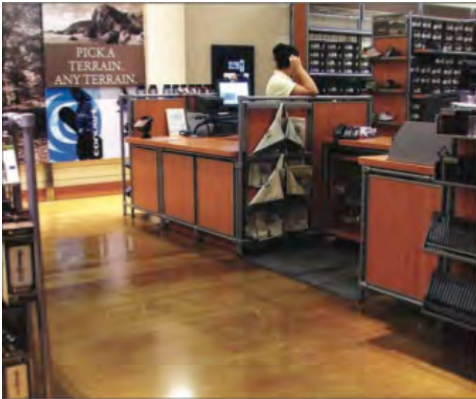
Polished concrete is not only easy to clean, but also creates a perception of cleanliness. This feature can be valuable,
