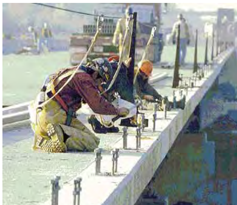
MetaMax® HRM used in high-performance concrete on dual four-lane bridges carrying I-87 over the Hudson River.
