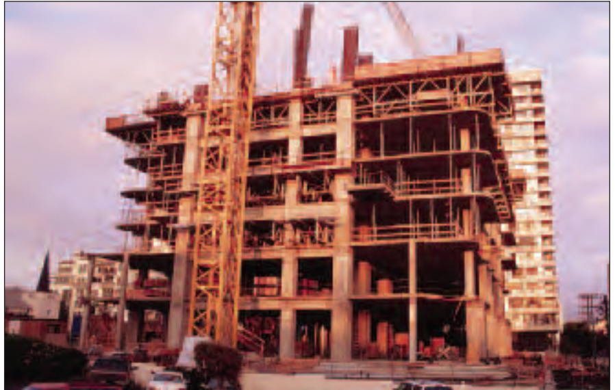
Late afternoon sunlight colors the lower floors of the structure, built with 12,000-psi concrete containing high-reactivity metakaolin. The large columns and beams of the moment frame, exposed at the center of the east and west facades, are in counterpoint to the minimal columns required around the rest of the building.
