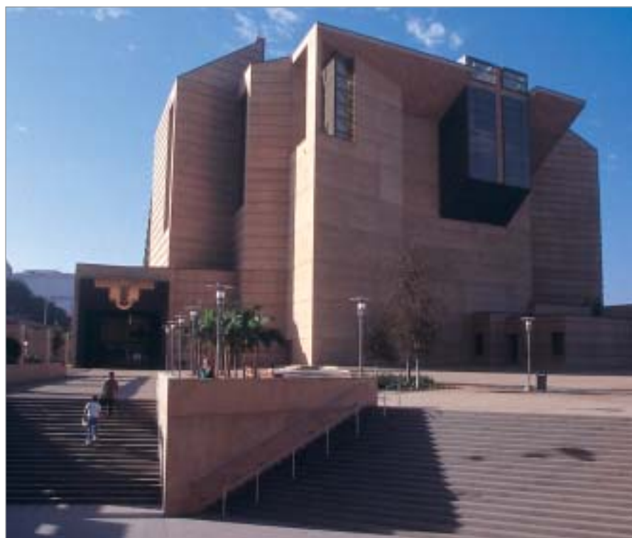
Sandblasting produced a roughened surface that scatters reflected light to soften the impact of mottling
