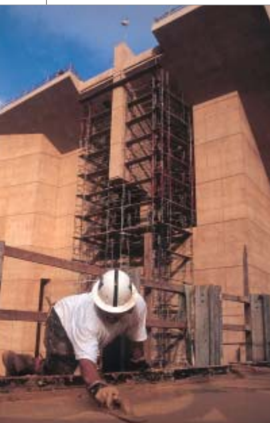
Sandblasting produced a roughened surface that scatters reflected light to soften the impact of mottling
